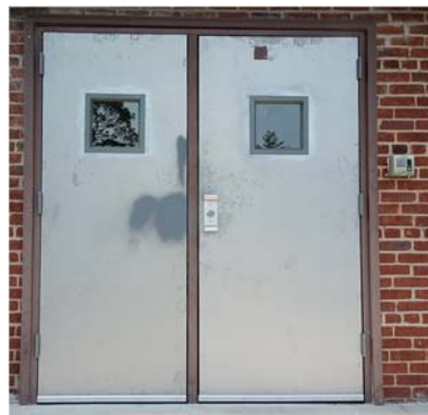
Sanctuary doors at top of handicapped access ramp.
